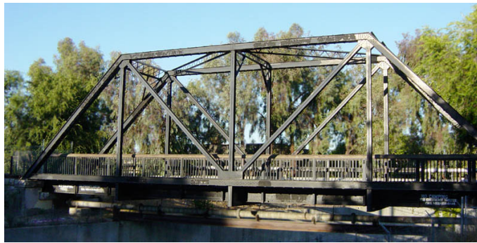
Figure 69 A simple truss
