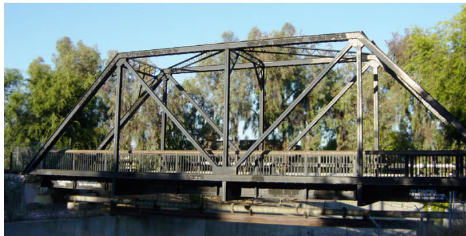
Figure 69 A simple truss
