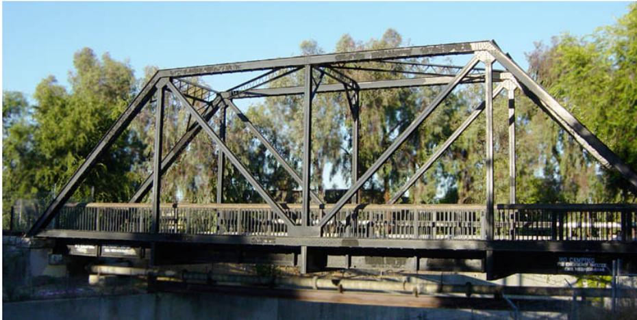
**Figure 69** A simple truss
